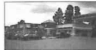
Appropriate. Combining two pad uses in an L-shape form helps to create an outdoor open space and break up the mass of the building.
